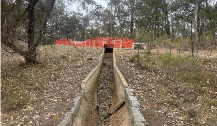
Failing infrastructure on the Specimen Hill Channel (photo: Melanie Tranter, Sequana)
