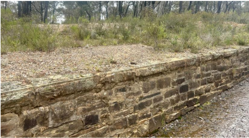
Bluestone lined channel near the Number 7 Reservoir (photo: Melanie Tranter, Sequana)
